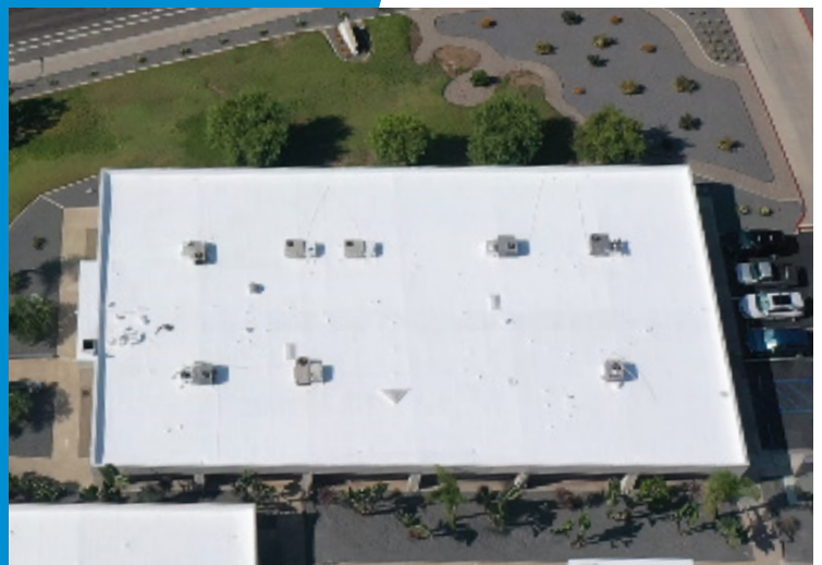
Auvil Fruit Company - Ultra-Thane 230 Spray Polyurethane Foam System Over Cold Storage
