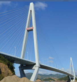
Taoyao men Bridge
